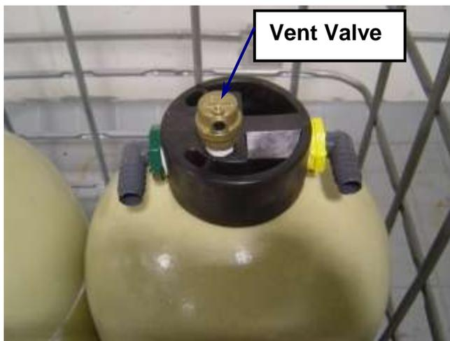
Figure 6: Filter Air Vent Valve
