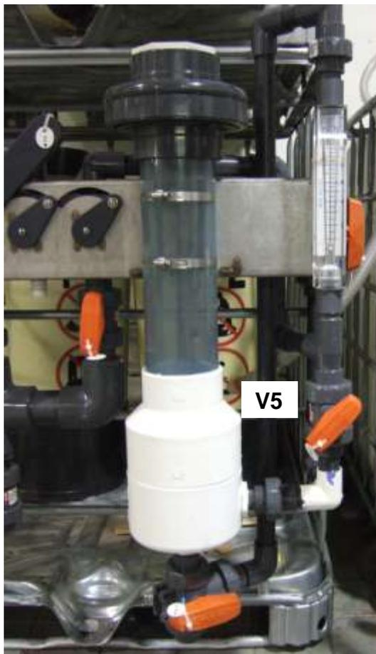
Figure 7: Chemical Feed Bypass Valve, V5, partially open
