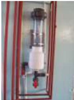
Picture of a chlorinator installed on well discharge line
