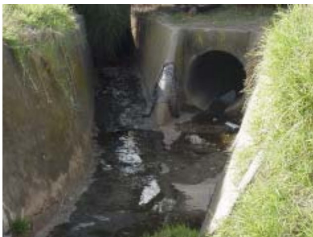
Figure 6 Site 01 flat cement drain
